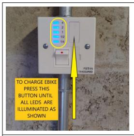
1) To charge your bike, press the button on the wall repeatedly until all 5 LEDs are lit. This will charge the battery for 4 hours – which is how long it takes for an empty battery to completely recharge
